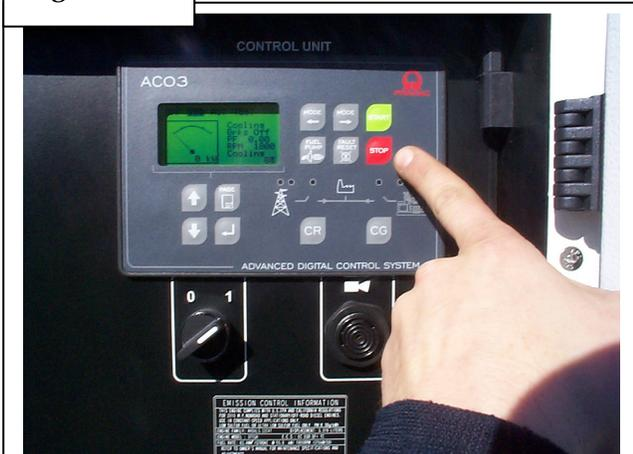
*Push the STOP button to initiate the stop sequence with cool down run time. Hold STOP button for immediate shutdown without cooling run time.*
